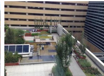
Intensive green roof at Lois Hole Alexandra Hospital, Edmonton, AB.
