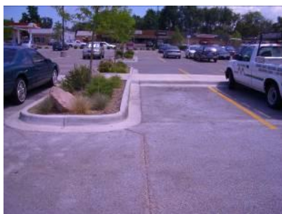
Porous Asphalt Parking Lot, Denver Photo Credit: AMEC Earth & Environment
