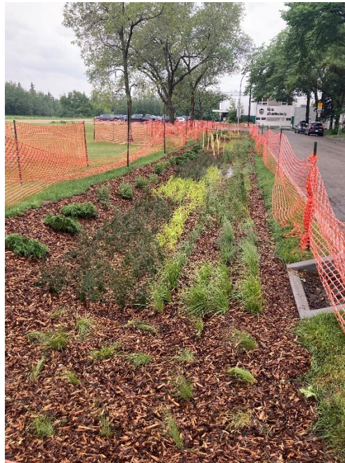
Shamrock-Donnan Park bioretention basin, Edmonton, AB.
