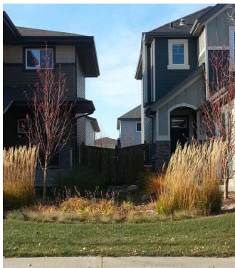
Residential rain garden installation.
