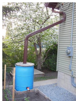
Residential rain barrel to harvest roof runoff for irrigating plants, Edmonton, AB.
