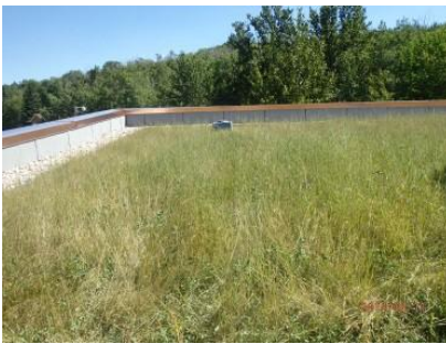
Green roof at Fort Edmonton Park Pump Station, Edmonton, AB.
