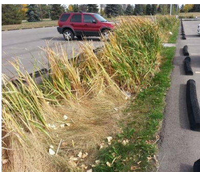
Bioswale at Mill Woods Parking Lot, Edmonton, AB
