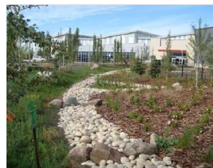
Bioswale at Terwillegar Recreation Centre, Edmonton, AB
