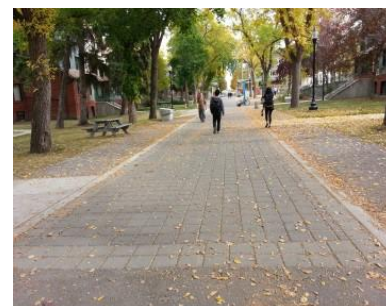
Permeable pavers walkway at the University of Alberta East Campus Village, Edmonton, AB.
