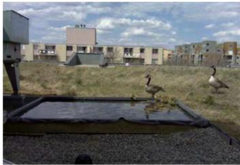
Downtown Building, Edmonton, AB.
